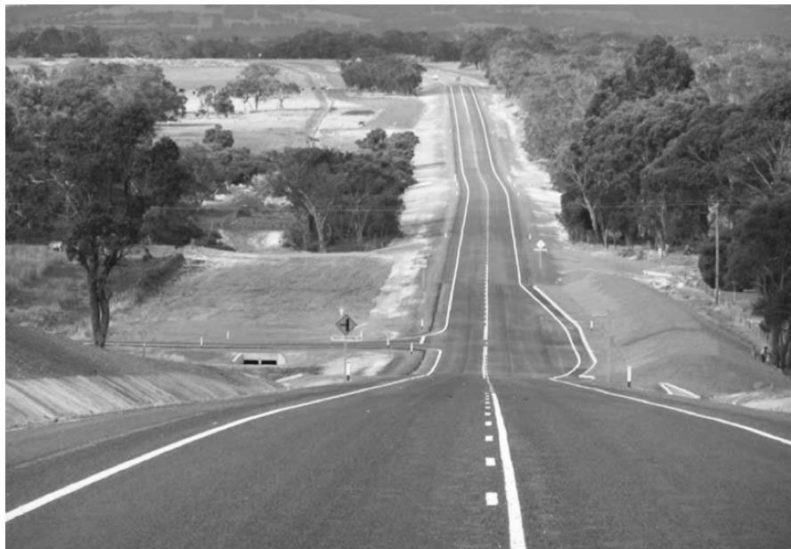
Stage 1: Constructed in 2007
